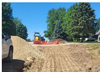
STORM SEWER TRENCHES COMPACTED WITH A SHEEPS FOOT STYLE COMPACTOR
