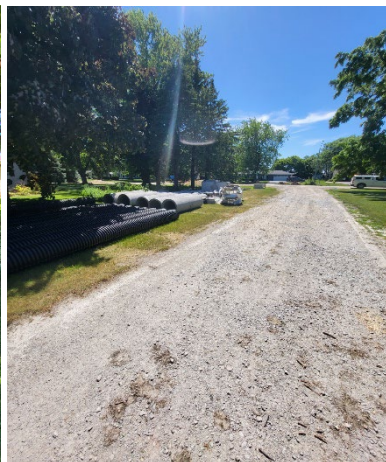
ALL STORM SEWER MATERIAL ONSITE, INSPECTED, AND APPROVED FOR INSTALL
