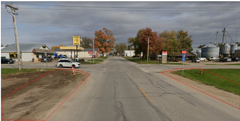
HWY 38 (Looking North at South Street)- Location of Stage 1 Construction
