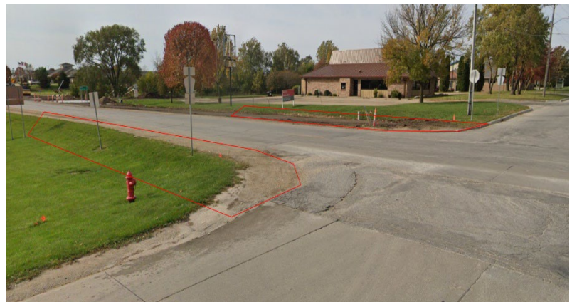
South Street (Looking Southwest at HWY 38)- Location of Stage 1 Construction
