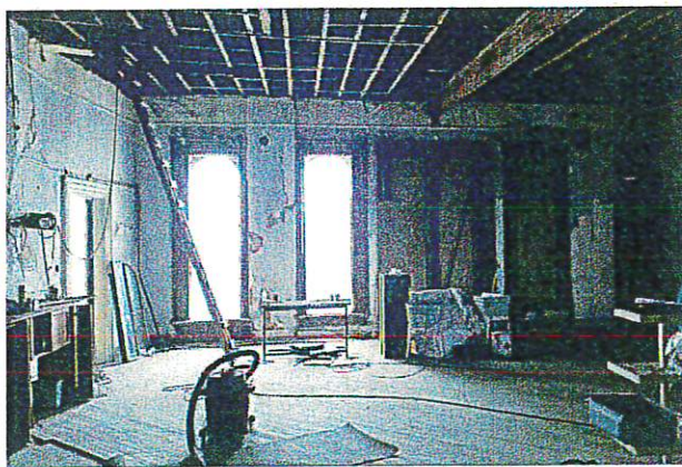
Photo 14 | Third Level, East Exterior Wall.
