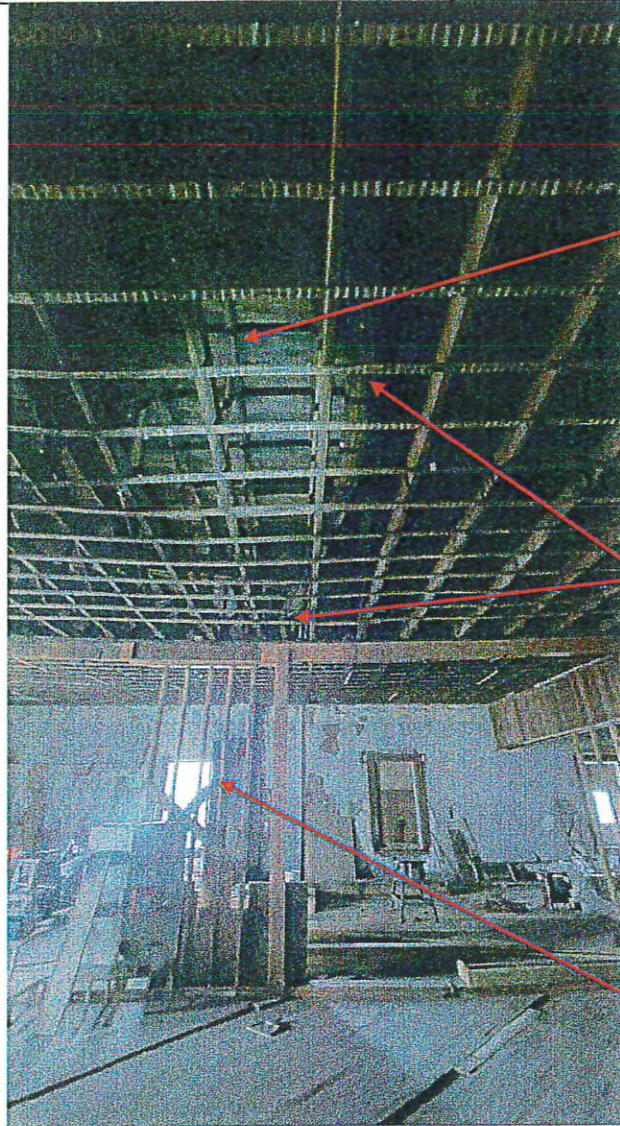
Photo 6 | Grid 4 Inverted King Post Truss, Looking South.
